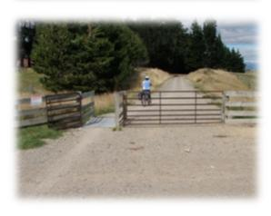
Grids are commonly used on rail trails at fence lines and property boundaries to prevent stock from escaping, but still allowing the passage of cyclists and walkers. This example is from the Otago Central Rail Trail in New Zealand. Similar examples can be found on the Brisbane Valley Rail Trail and the High Country Rail Trail in Northern Victoria.
