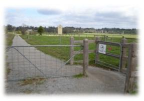
The gating system at road crossings used on the Lilydale Warburton Rail Trail in Victoria makes it difficult for unauthorised users (such as motor bikes and 4WD vehicles) to gain access to the rail trail.
